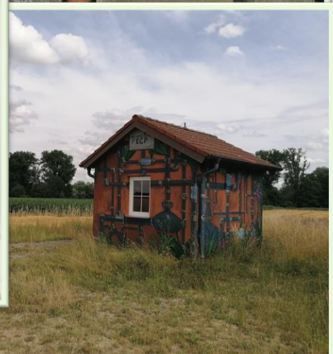
Pumpstation am Wasenhof
